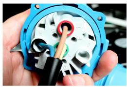
**Step 8:** Position the leads of the new cord in the existing plug. Tighten to 15 inch-pounds of torque.
